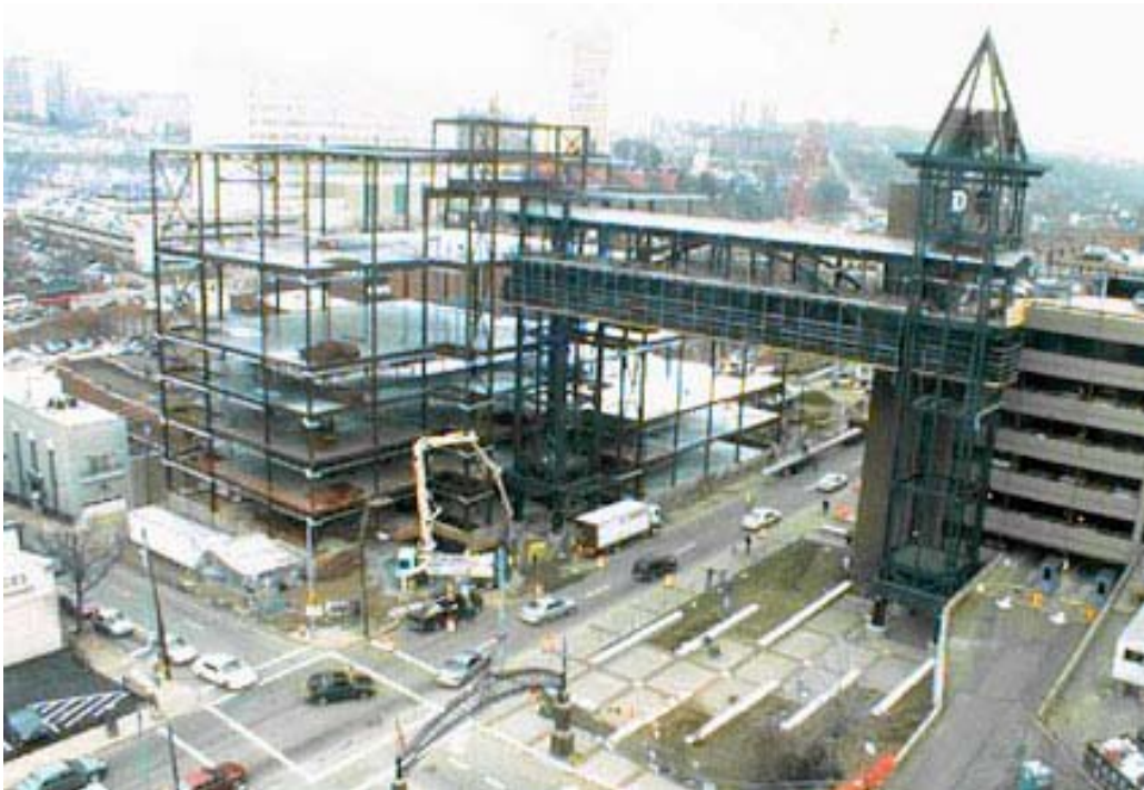
Construction as of November 2006
